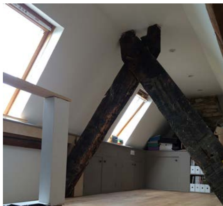
The cruck beam
